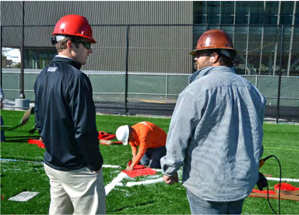
Jimmy Francis (left), Director of the Student Recreational Center and Cory Hughes (right), a FieldTurf foreman, talk about the progress of the turf field, while Mauricio De La Cruz (middle), a FieldTurf installer, glues together the softball home plate. Photo credit: John Saringo-Rodriguez / Daily Sundial
