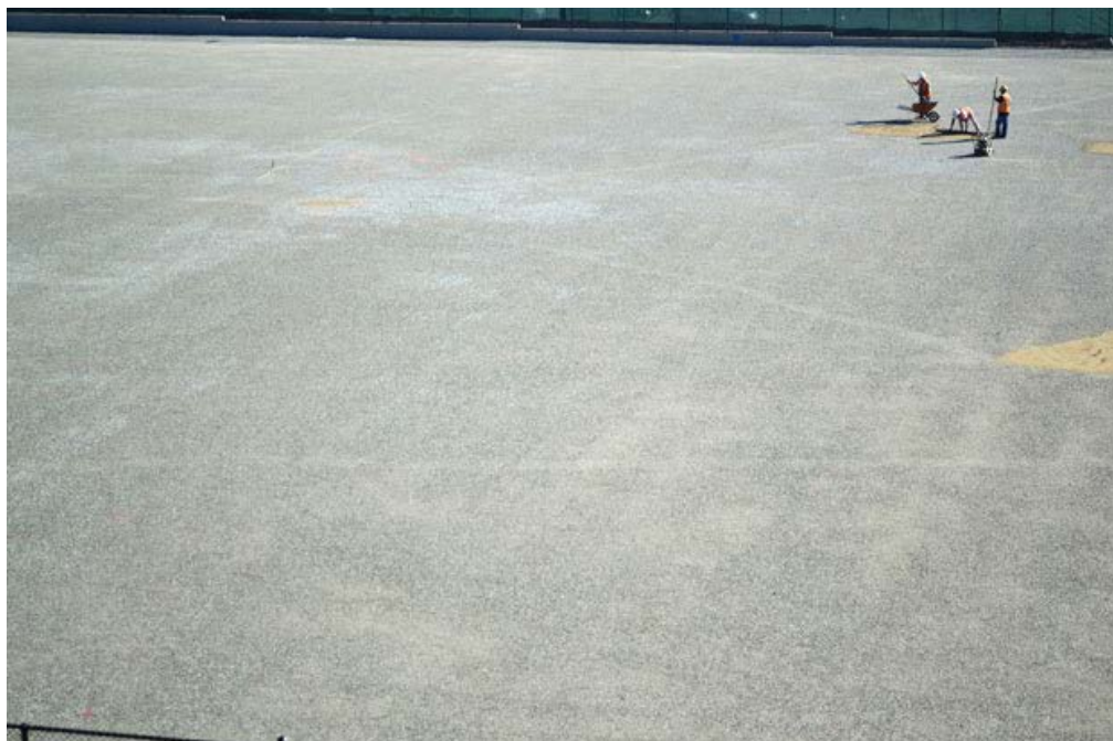
OHNO construction workers make sure that gravel is consistently flat and level before the grass can be placed on the field. Photo credit: John Saringo-Rodriguez / Daily Sundial
