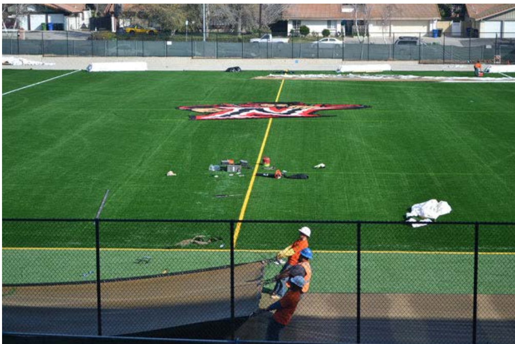
FieldTurf construction workers drag the polyurethane grass across the side of the main field. Photo credit: John Saringo-Rodriguez / Daily Sundial
